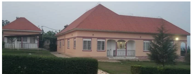
Behind view showing worker`s house.
